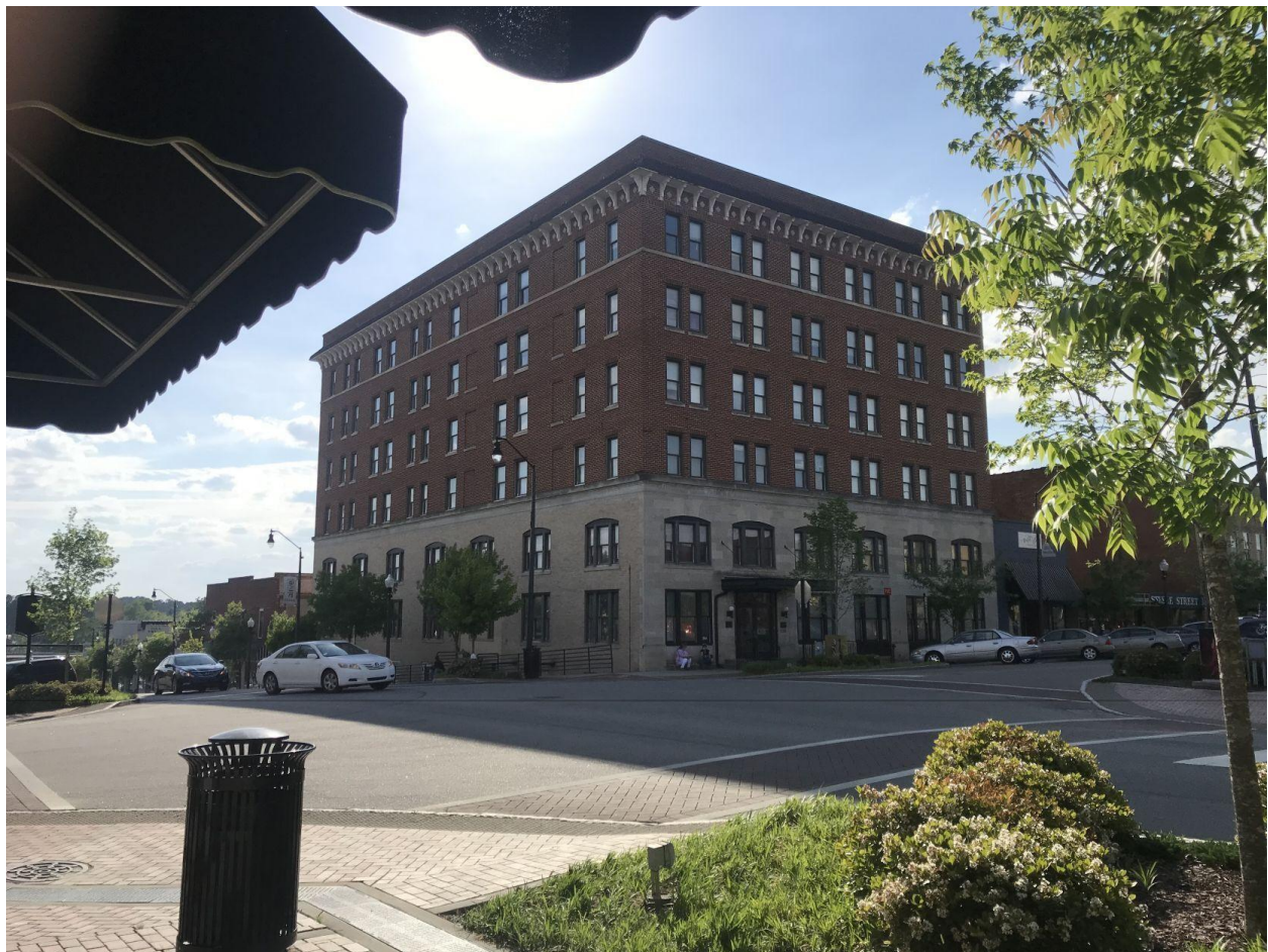
Wilrik Apartments, on South Steele Street, is an affordable housing building the Sanford City Council is considering improving with American Rescue Plan funds.
